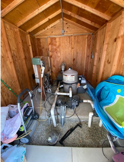
INTERIOR OF SHED
